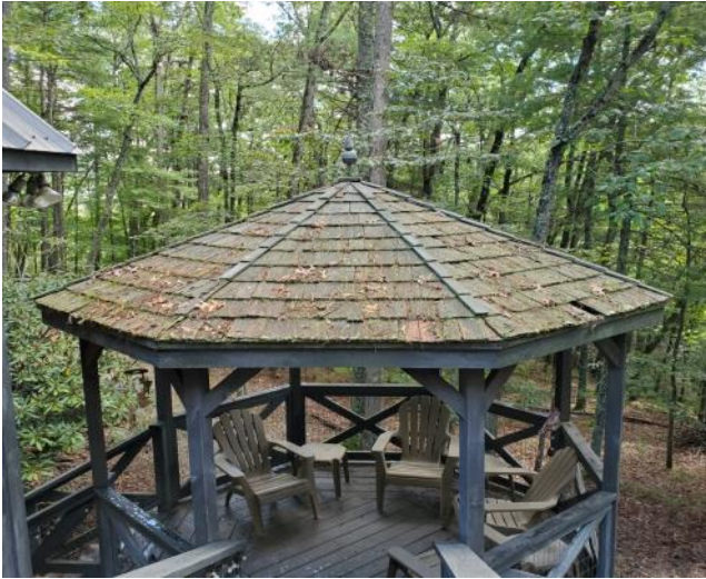
BEFORE: Gazebo (aka Silo) —Cedar Shake Roof needed replacing
